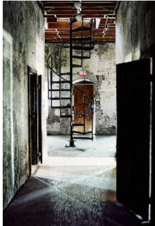
The old Charleston jail, which retains many 19th-century features including this iron staircase, provides a working laboratory for students, and classroom and office space.
